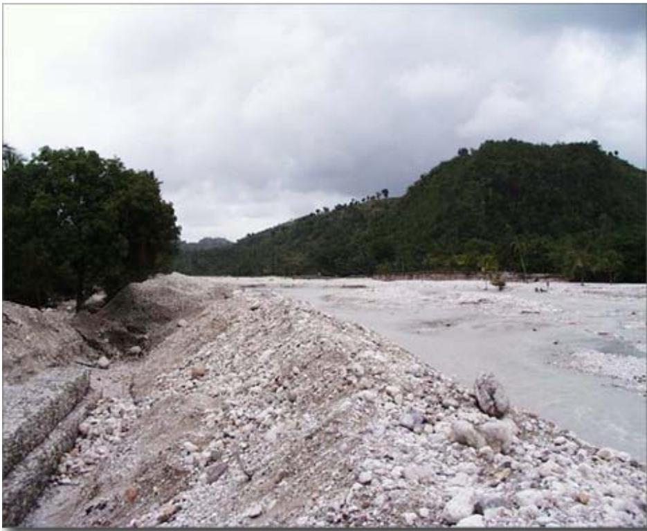
This photo, taken two weeks before the floods, shows the dyke construction (on the left) designed to keep the river within its banks. The main road is hidden to the extreme left
